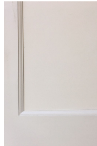
Detail, stile and rail, recessed panel and bead
